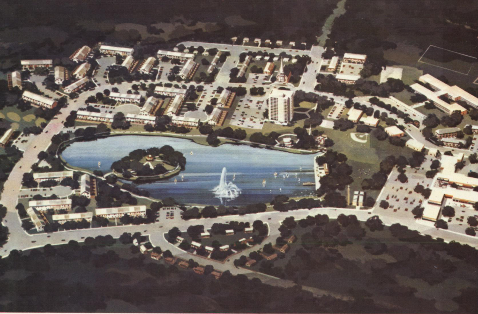
Belair Village, one of the latest developments in modern housing, was opened in September 1968 in Prince Georges, Maryland by ITT's Levitt & Sons, Inc. This planned-for-living community for 30,000 residents has 200 acres for recreational use, including a children's zoo and a lake at the town's center for boating, fishing, and swimming.
