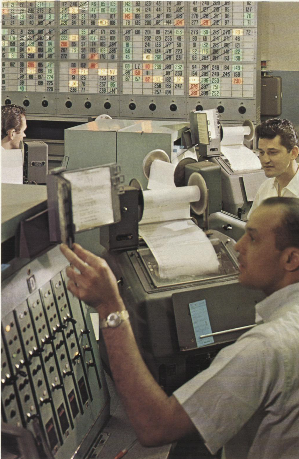
Left: Advanced equipment such as the electromechanical trunk display board in background enables telex operators at ITT World Communications New York headquarters to obtain up-to-the-minute status of radiotelegraph circuits in the company's global network.
