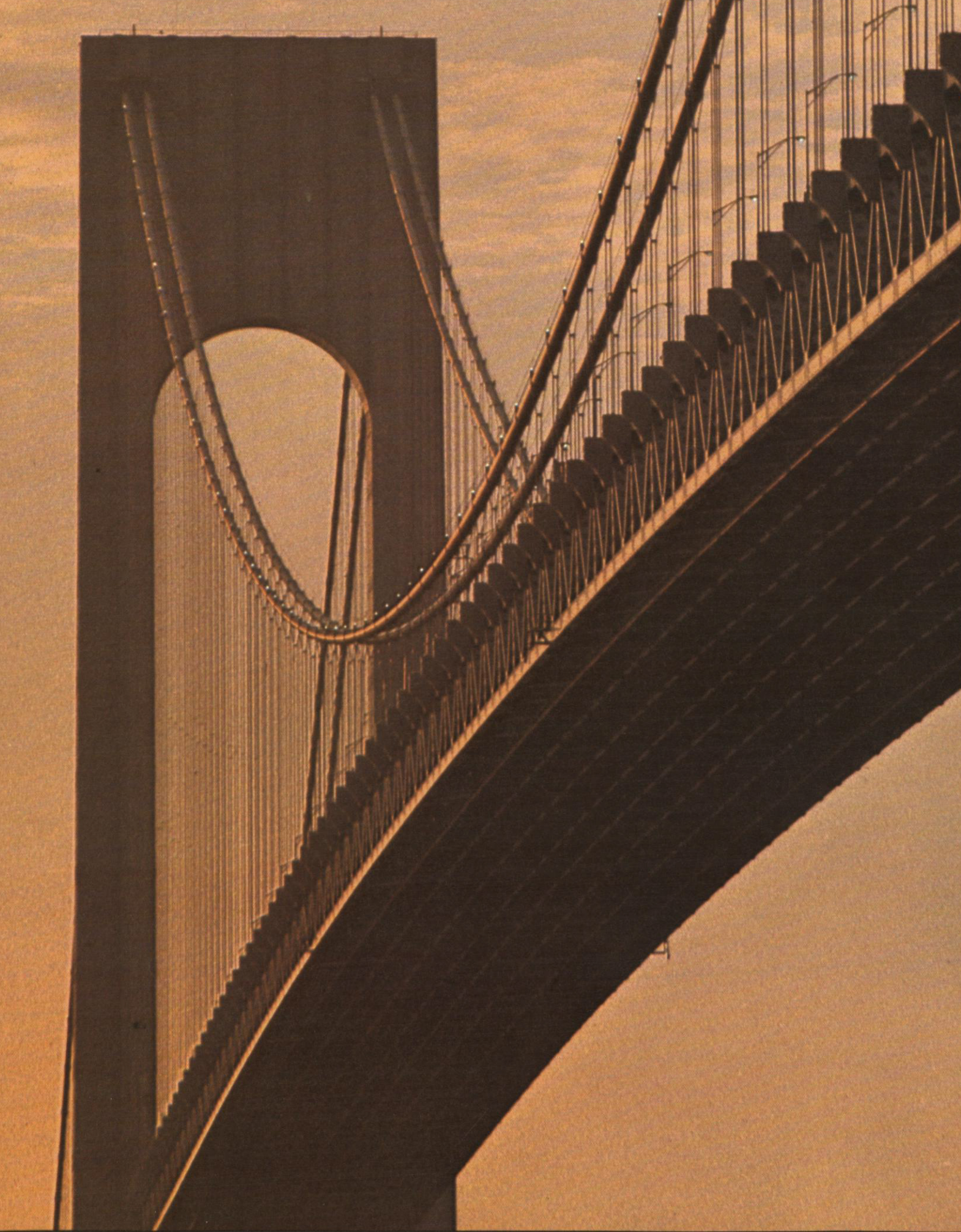
More than 2,300 tons of special high grade zinc from G+W's metals and chemicals group were used to galvanize the main cables of
