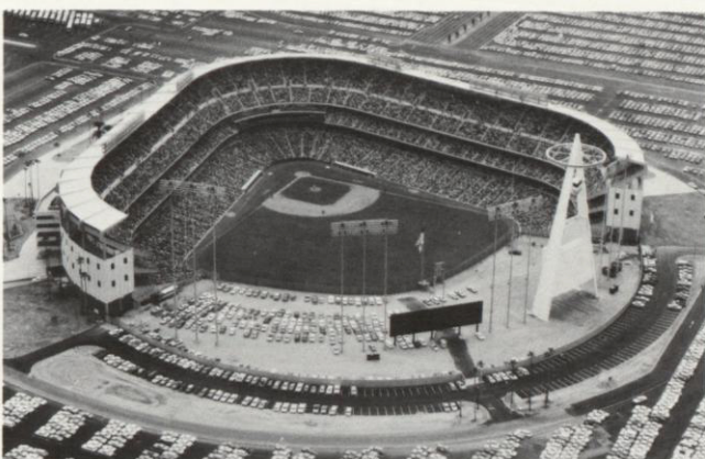
Anaheim Stadium, home of the Angels, has been provided with one of the finest sound systems ever engineered for an outdoor ballpark by LTV Ling Altec. Behind center field, the 90-foot tower depicted here provides absolutely clear sound over a distance of more than 700 feet to blanket the entire ballpark.
