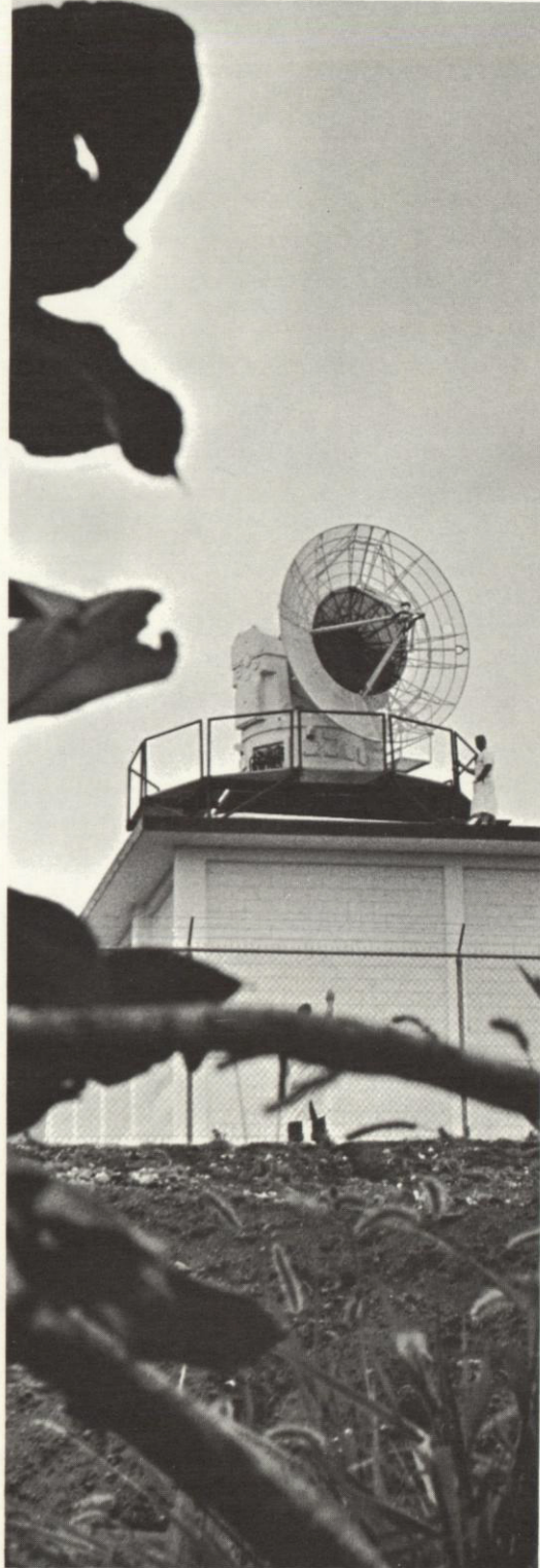
The tracking antennas at LTV's Hawaiian Mercury Tracking Stations keep in constant contact with the astronauts as they orbit across the Pacific.
