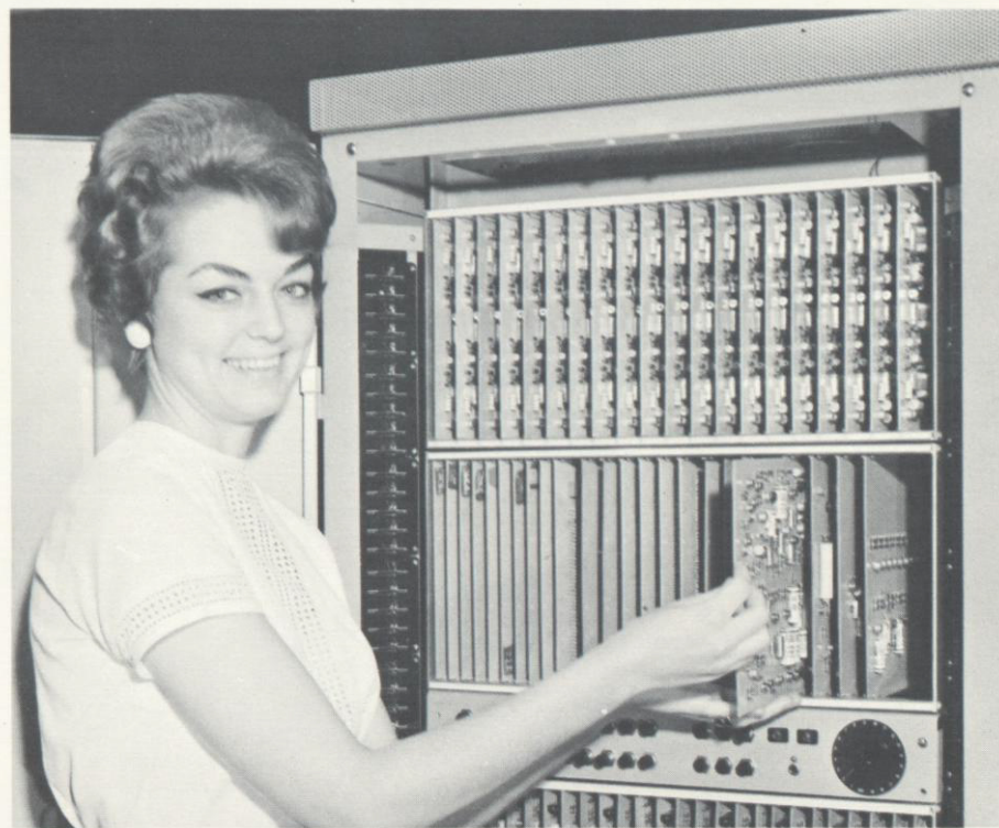
Above, world's largest trunk telephone exchange located in London and equipped with switching apparatus made by one of our English companies. Below, new ITT electronic private automatic telephone exchange made in the United States. Light on panel shown in photo indicates where to replace circuit board.
