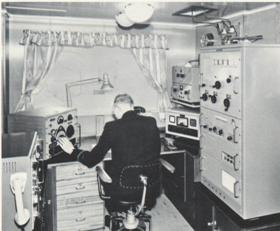
Top photo shows part of new automatic switching equipment installed during 1962 in New York headquarters of ITT's worldwide cable and radio communication system. Below, view of radio station aboard a Norwegian cargo ship. ITT equipment includes a combined teleg-raphy-telephony transmitter.
