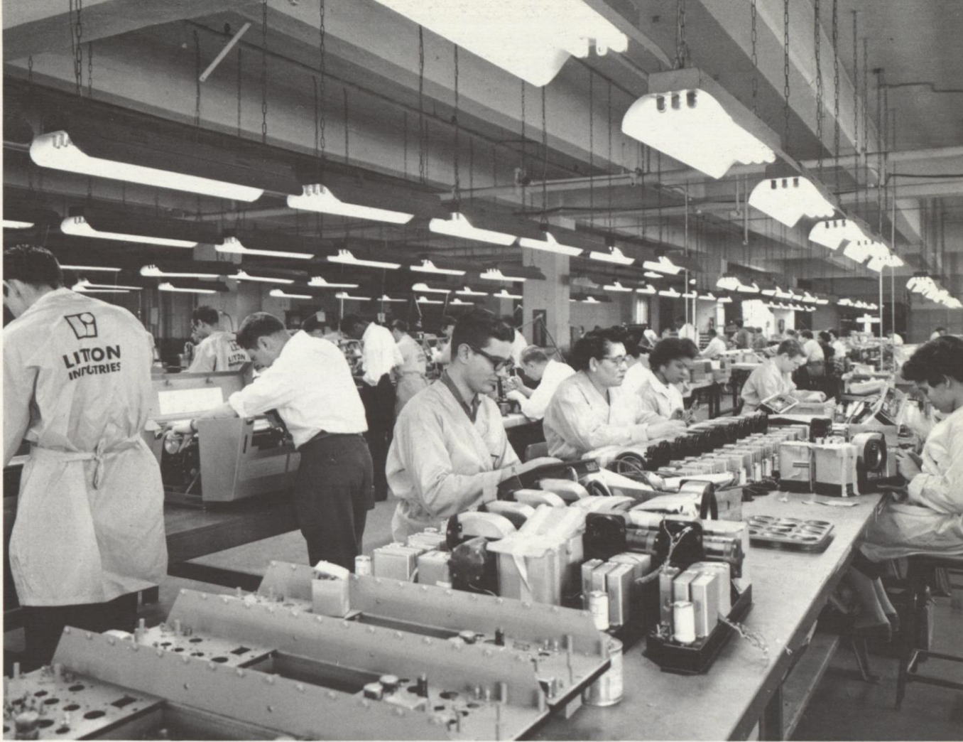
FACSIMILE COMMUNICATIONS EQUIPMENT FOR MILITARY AND COMMERCIAL USE IS ASSEMBLED AT THE WESTREX CORPORATION DIVISION'S NEW YORK PLANT
