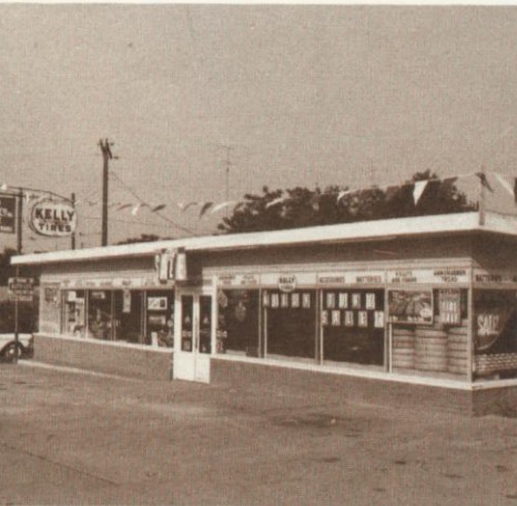
Representative of the Wood Tire & Supply Company operation is this store in Palestine.
