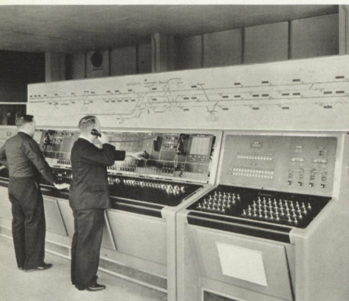
Operators follow train movements on track diagram of train-describer equipment produced by ITT System in England and installed in Midland Region of British Railways.
