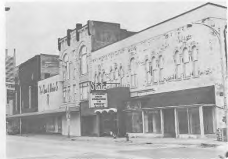
Tall stone building at the left (west) of the State Theater was the home of Rockford National Bank before the Rockford Trust Building was built.
