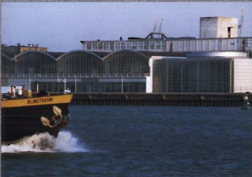
Overlooking one of Europe's busiest waterways, the new building of MarineSafety Rotterdam is physically positioned, and extensively equipped, to establish the highest levels yet achieved in the training of nautical personnel, ranging from ship's crewmembers, tugboat captains up to port traffic control operators and port officers. A joint venture with the Municipality of Rotterdam, the MarineSafety center accommodates five bridge simulators and one vessel traffic services simulator. The full mission bridge simulator features a wheelhouse on a motion-base surrounded by a 360 degree computer generated visual system. With its realistic sound and vibration simulations and depth of software, it is the most advanced maritime training device in the world.
