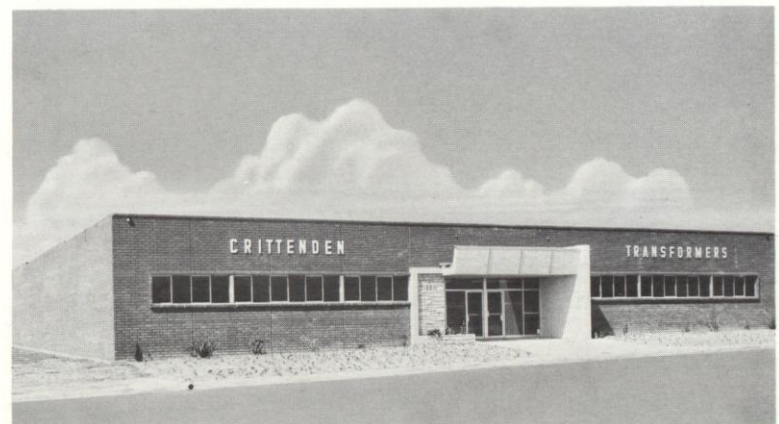
Crittenden Transformer Division in Los Angeles.
