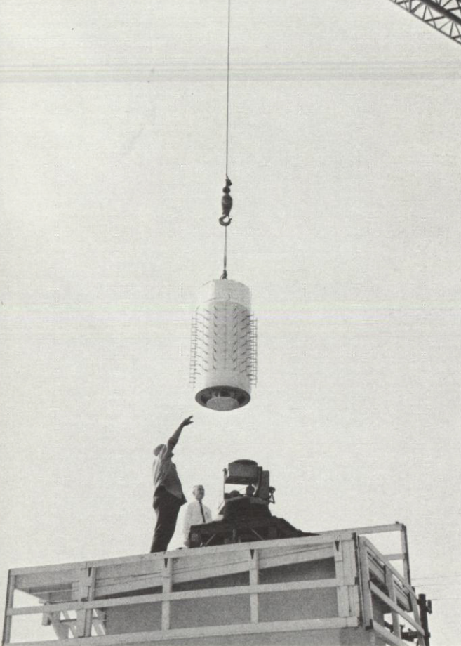
Experimental antenna for ground Tacan navigation stations, shown during installation on the Teledyne pattern measurement range. This cylindrical phased array is designed to provide improved coverage over a greater volume of space.
