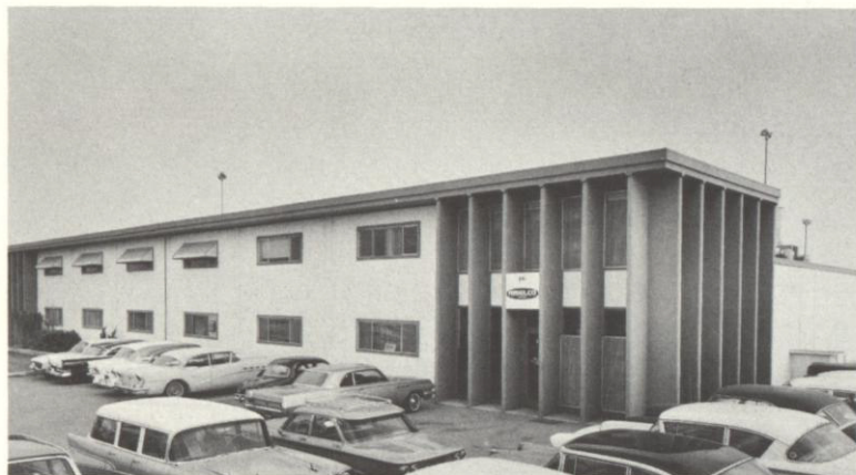
Existing plant of Electron Devices Division in Mountain View.
