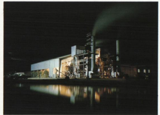
Waste wood boiler.
