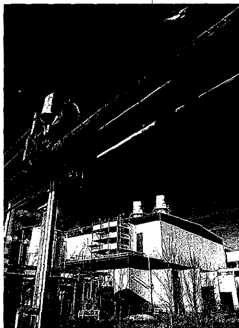
The Saranac gas-fired cogeneration project located in Plattsburgh, New York sells electricity to a utility and also natural gas through the Company's North Country Gas Pipeline.
