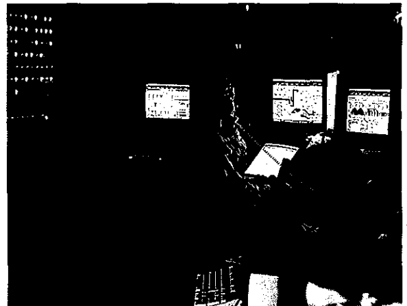
Consolidating Imperial Valley's control room operations enables the operators to efficiently monitor several geothermal power projects at one time.
