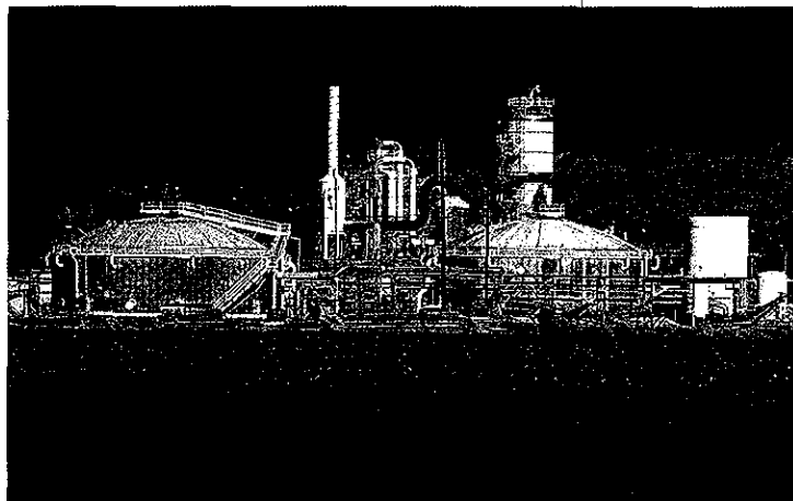
The Leathers power project produces electricity solely from naturally occurring geothermal steam near the Salton Sea Known Geothermal Resource Area in Southern California's Imperial Valley.
