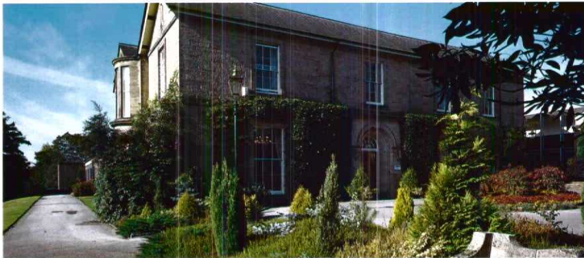
European research and development, testing and marketing are based at this Lubrizol facility in Hazelwood, England.
