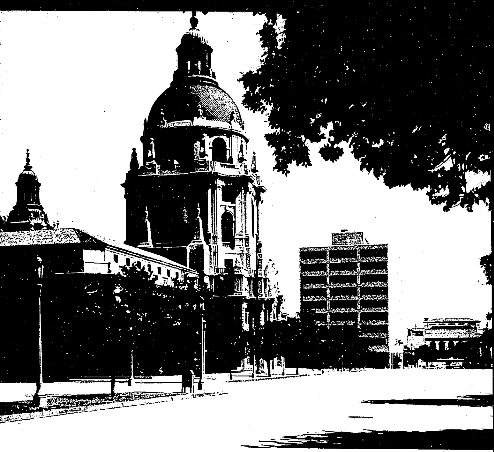
Headquarters building of Wesco Financial Corporation and Mutual Savings — Pasadena's City Hall in foreground
