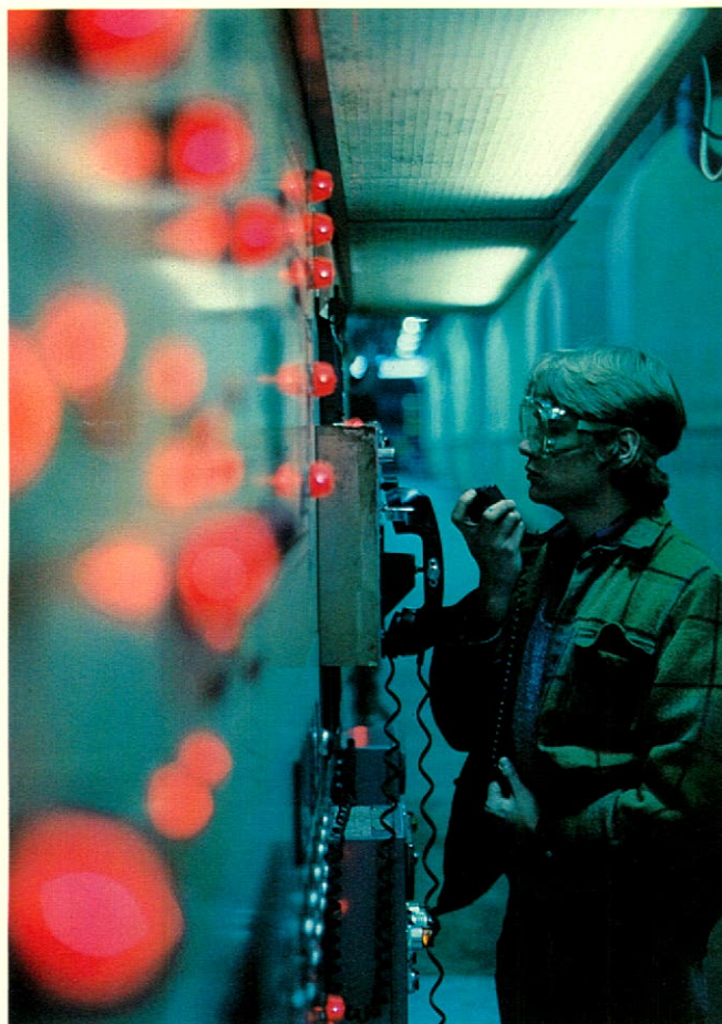
Checking the "nerve center" of a fiber glass mat machine; virtually all electrical circuits are monitored from this panel, which controls the entire mat manufacturing process.
