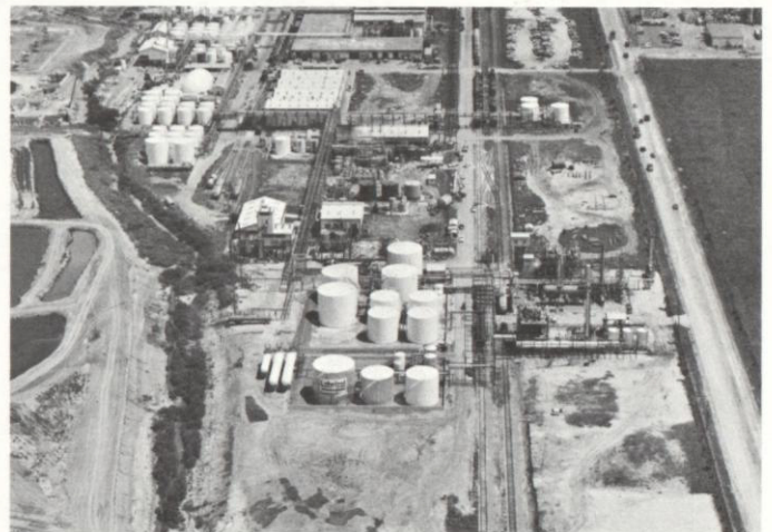
The Deer Park, Texas plant was further expanded in 1968.
