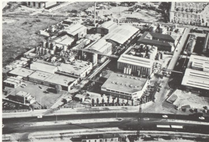
Lubrizol's plant at Rouen, France, is the company's largest manufacturing facility overseas.
