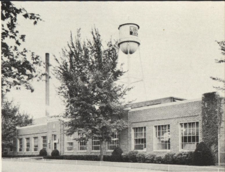
The Mechanical Testing Laboratory
