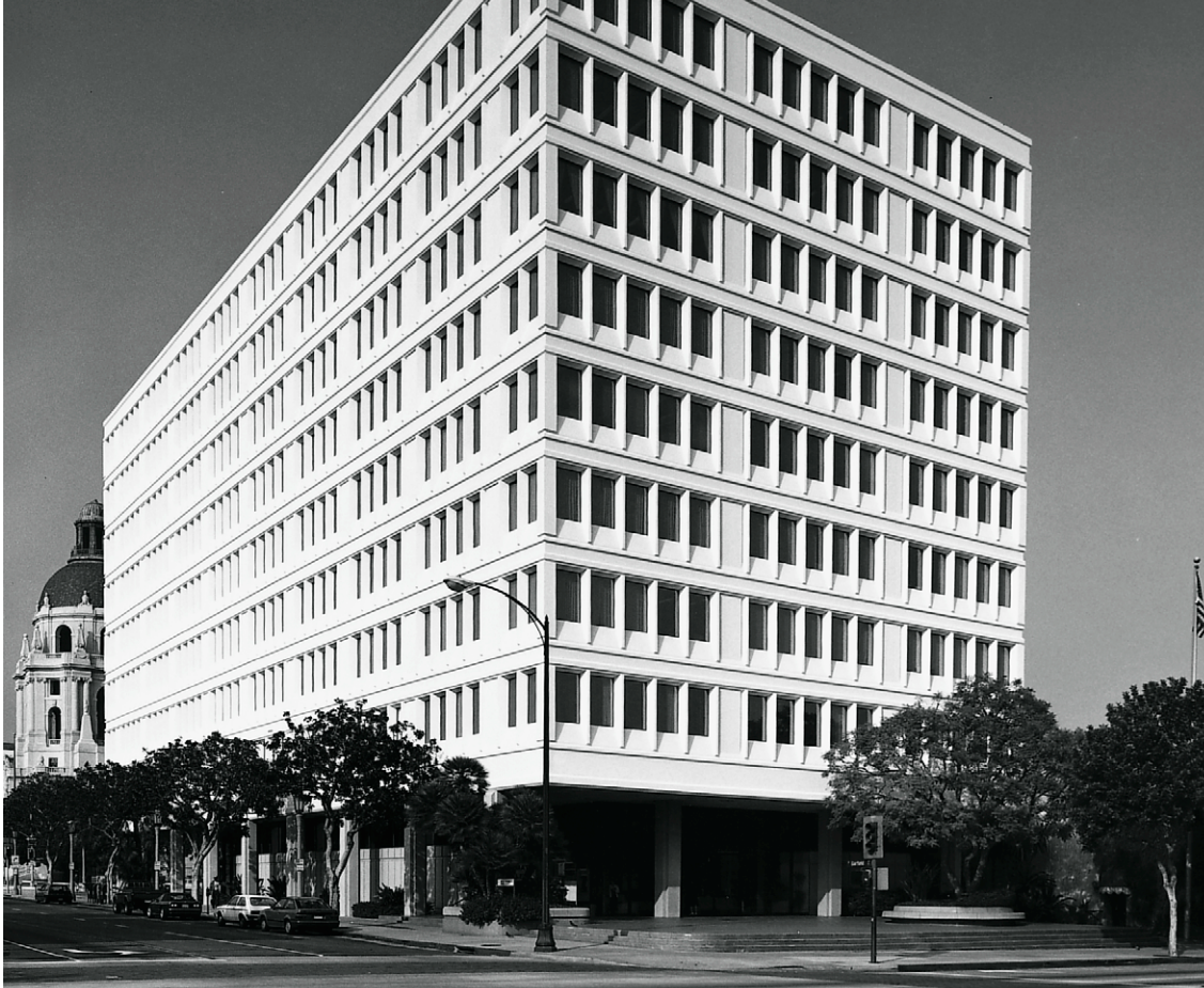
Office building owned by Wesco's property subsidiary, with Pasadena city hall in the background
